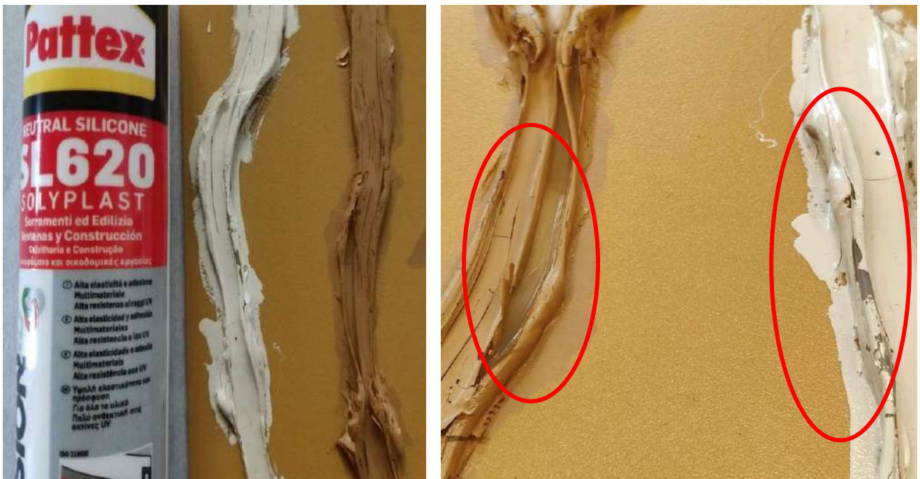
Figure 20-21: Touch-Up paint detachment on non-paintable silicone
