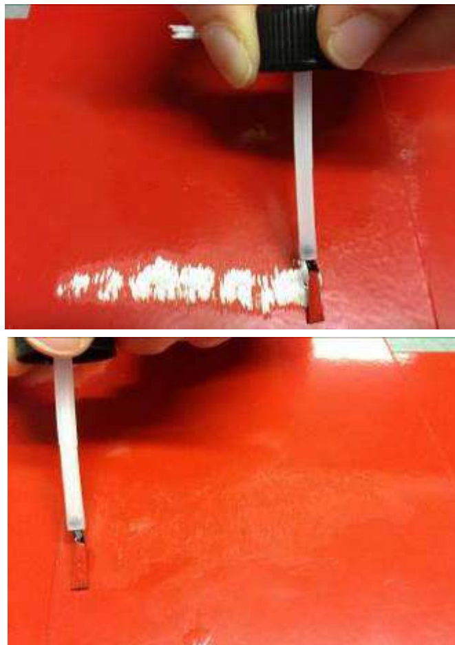
Figure 1-2: Application of the touch-up paint (before and after)
