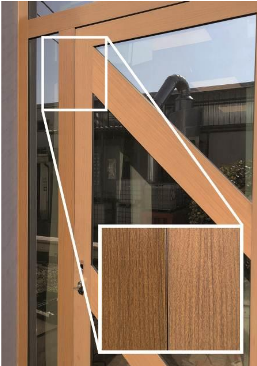
Figure 4: Door PARTIALLY cleaned
